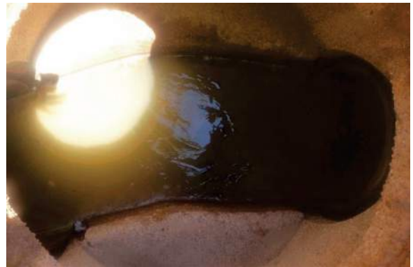
Manhole Before Install
