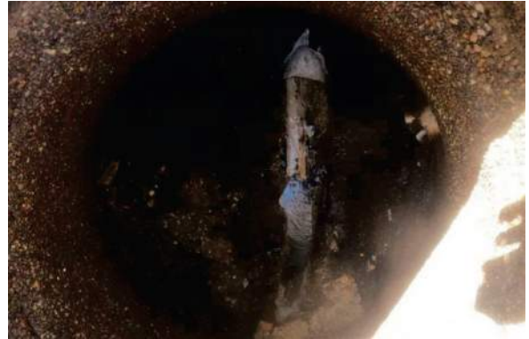
Manhole Before Install
