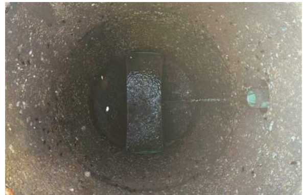
Manhole Before Install
