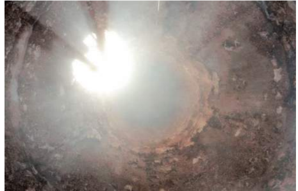
Manhole Before Install
