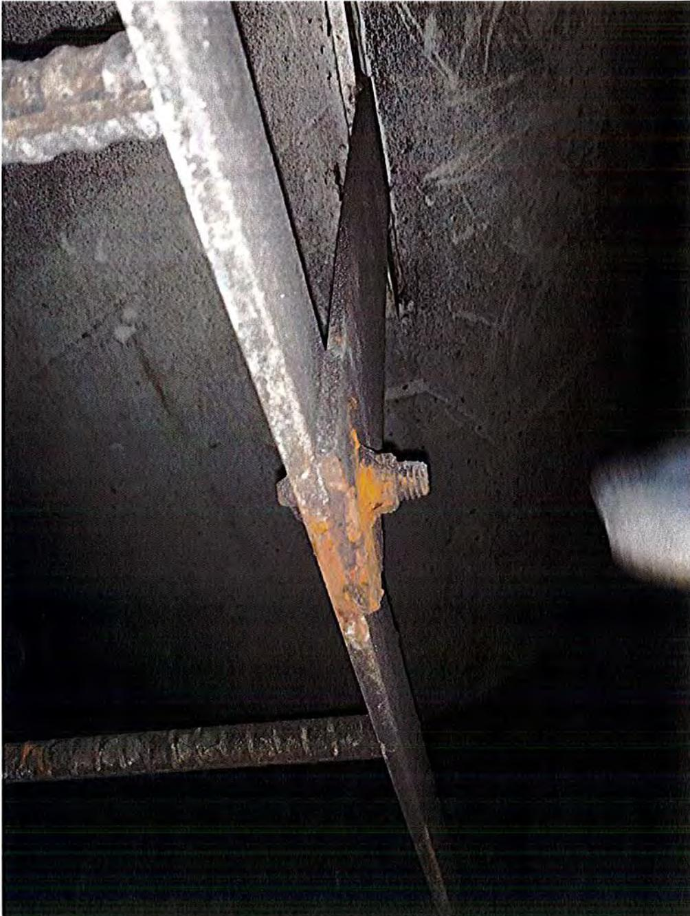
Bolt Corrosion on Interior Ladder
