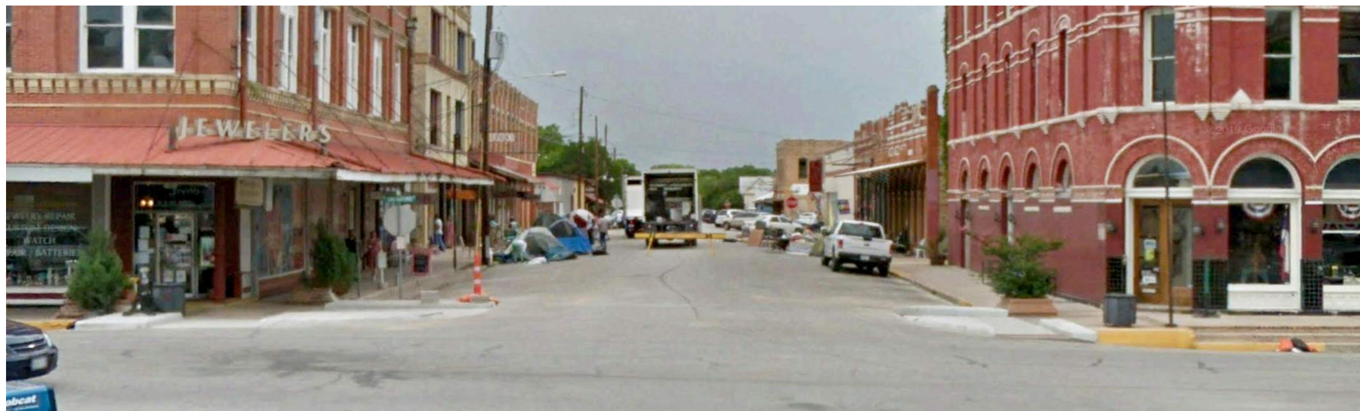
SAN ANTONIO + MAIN LOOKING NORTH
