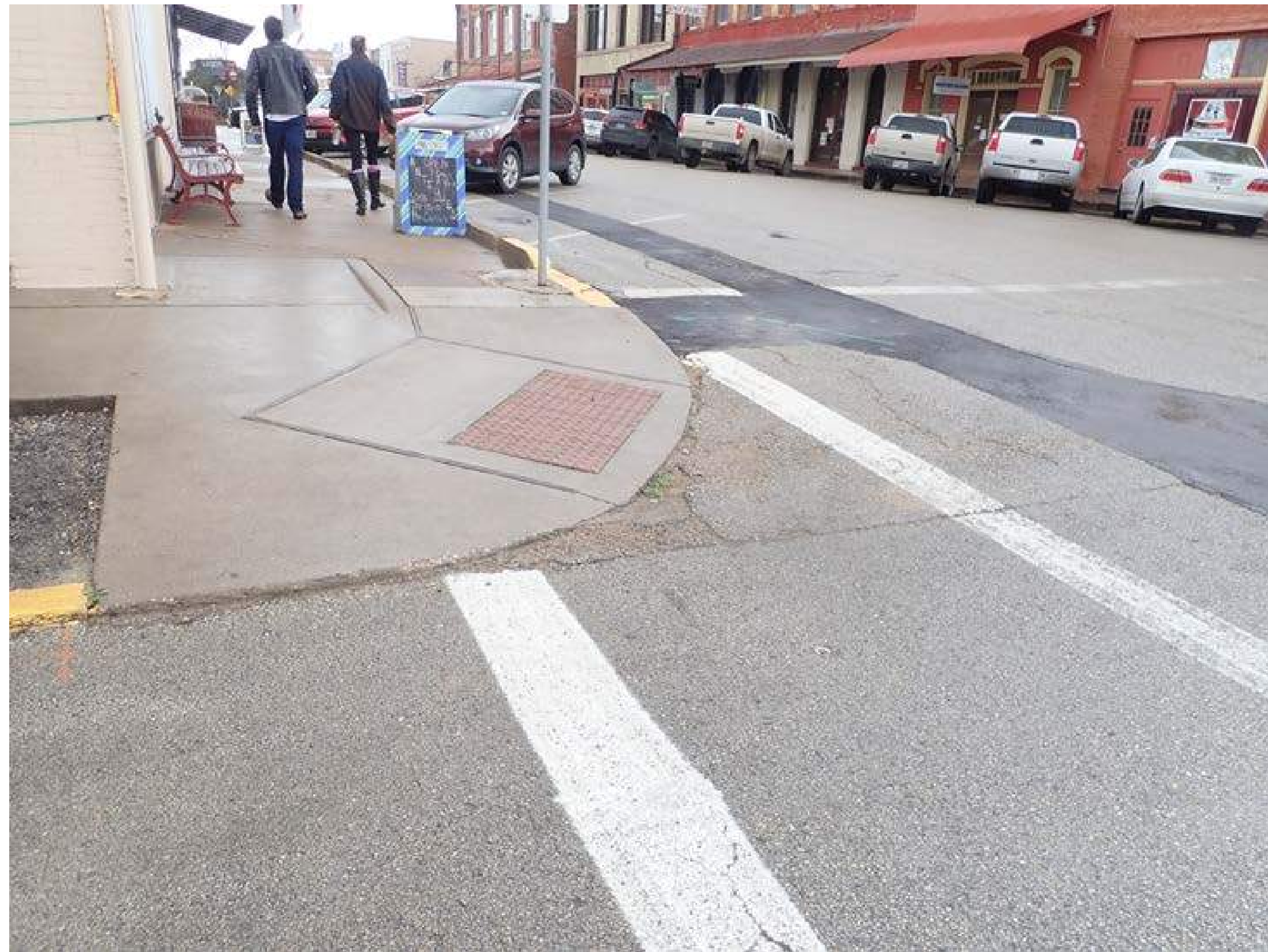
N Main St at Walnut - Looking South
