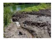
Runoff from bridge construction area observed entering Oso Creek
