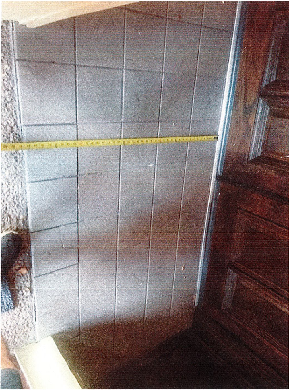
Photo of 105 S. Colorado Street side for tile replacement
