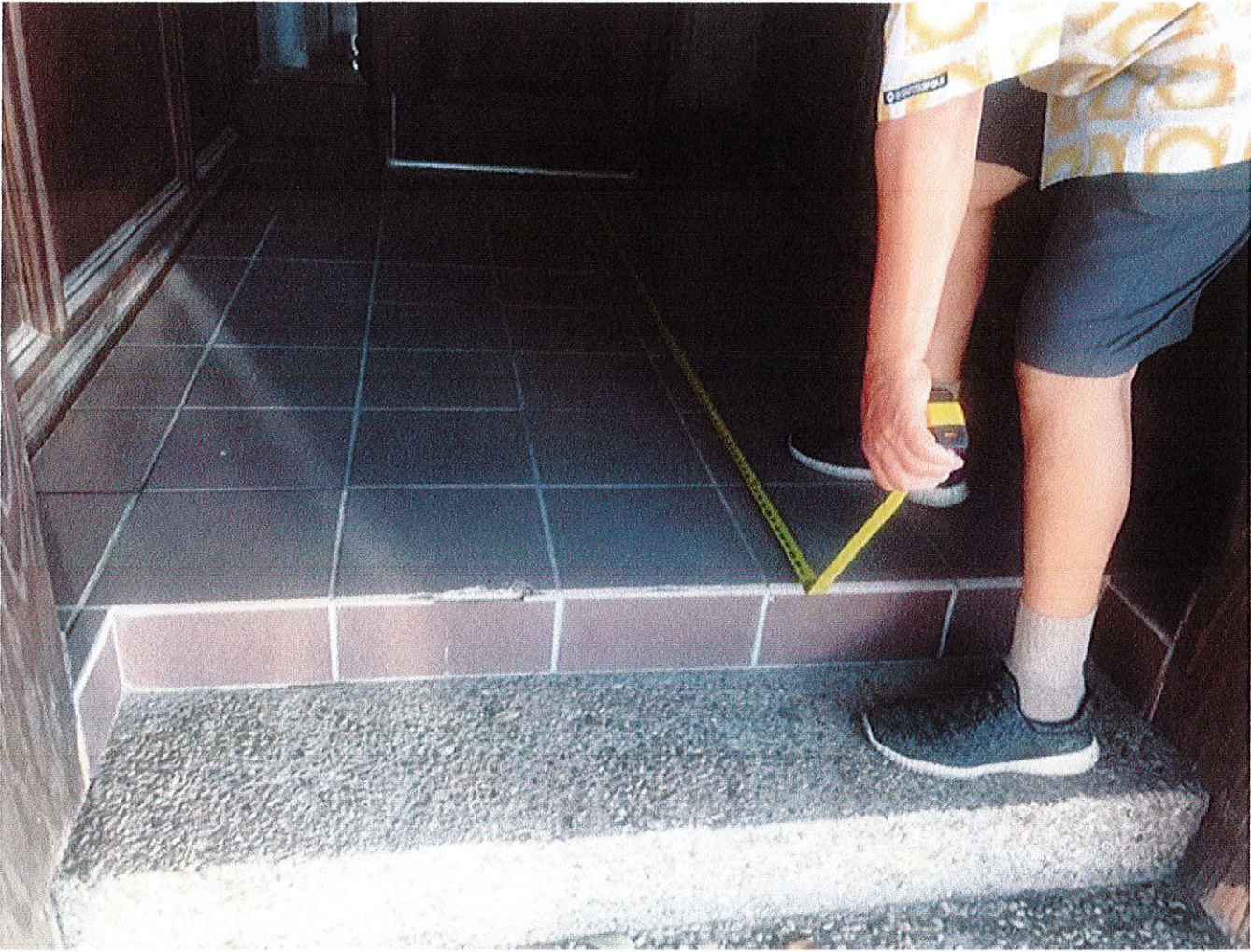
Photo of the 215 Market Street side for tile replacement
