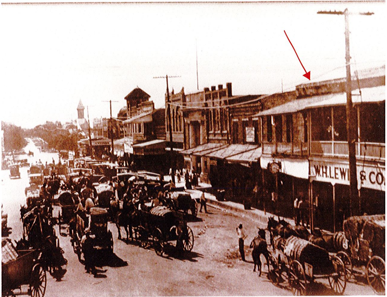
West side of Square, looking south, W. H. Lewis & Co., 1915-1925 Shows roofed balcony
