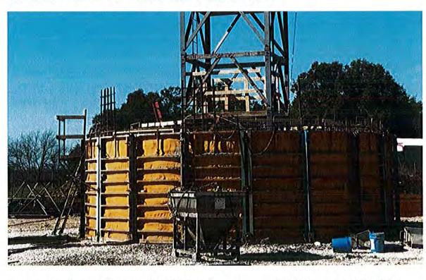
Contractors have begun work on the base of the new 500,000-gallon elevated water storage tank at FM 2001 and SH 130.
